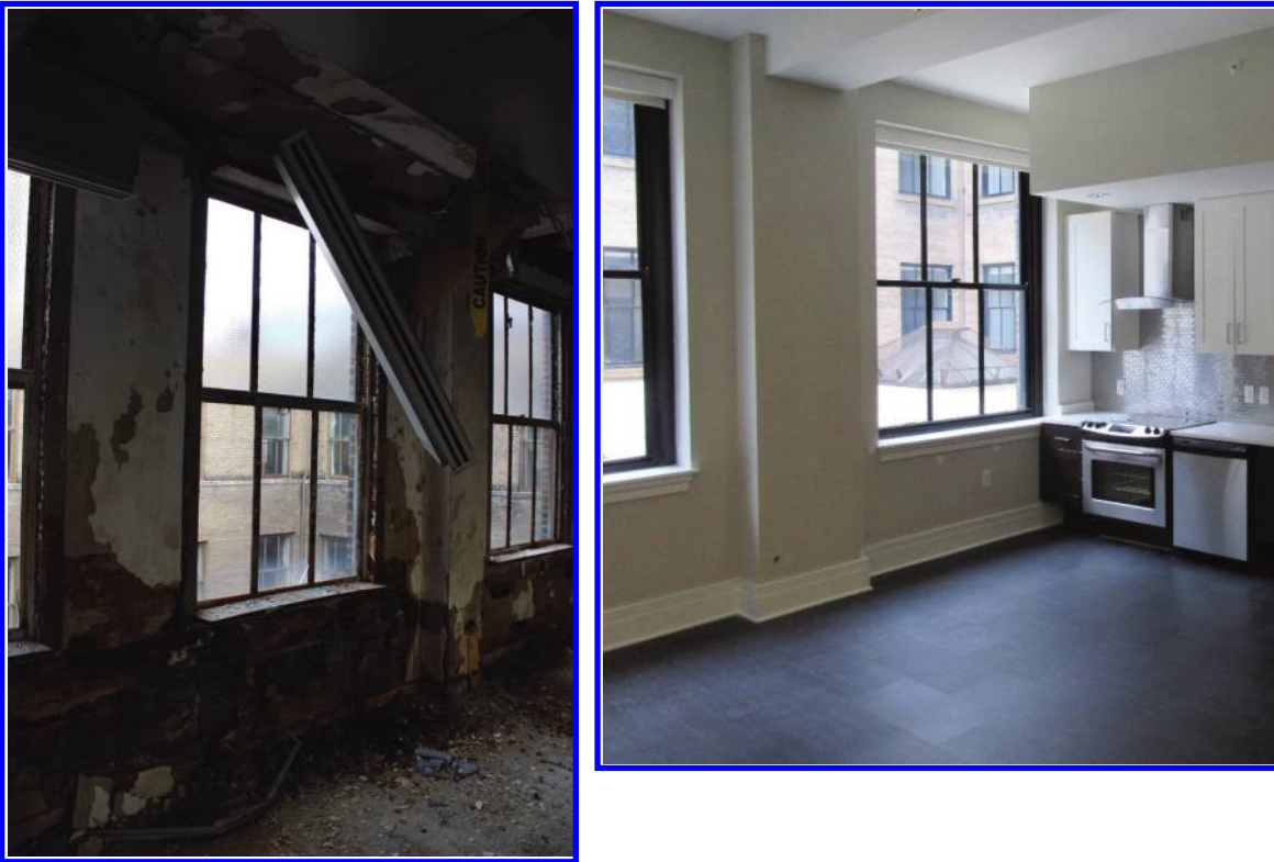
FIGURE 17: Before and after photos of Annex walls w/ insulated metal stud and gypsum board furring and refurbished steel windows
