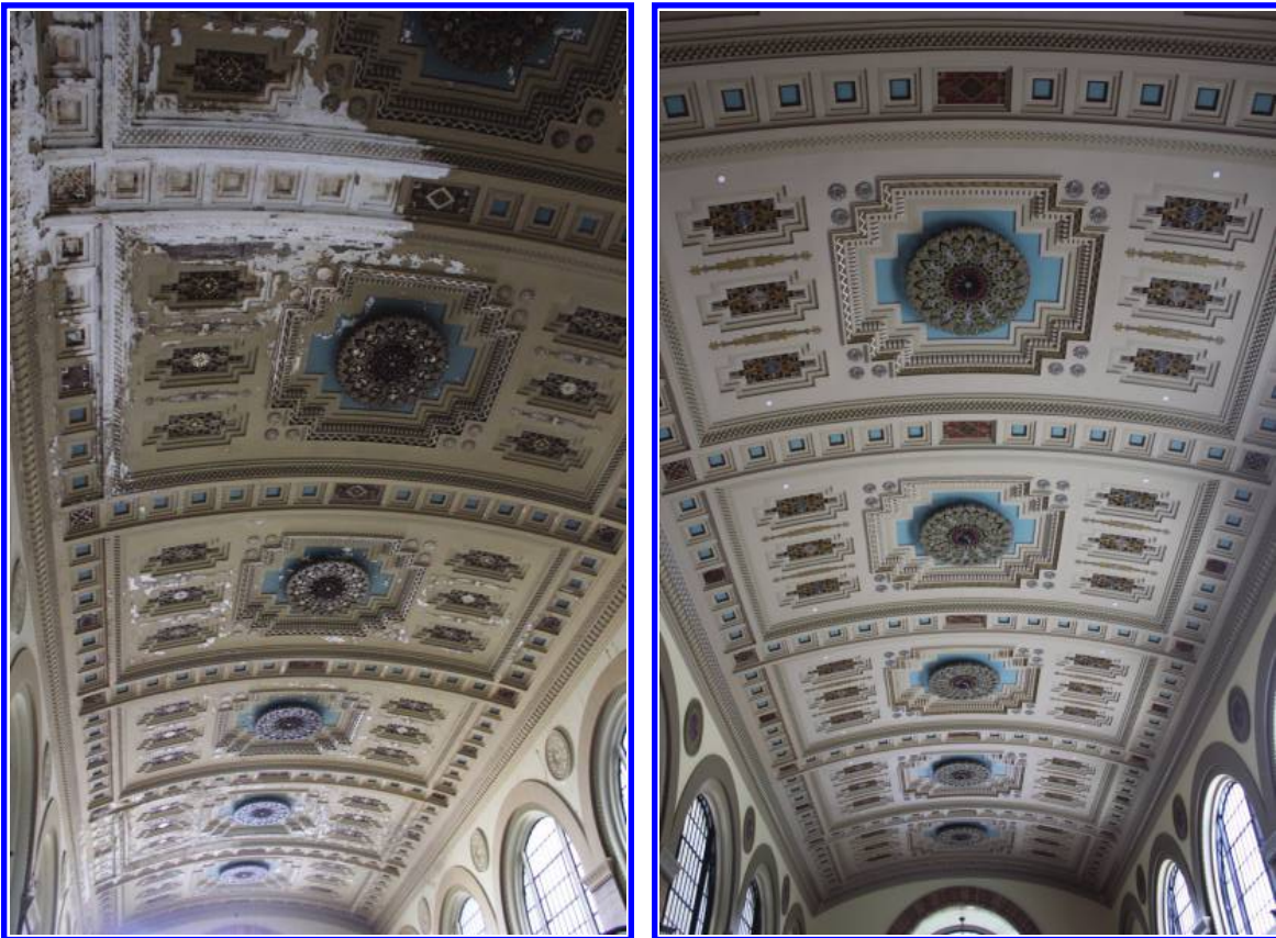
FIGURE 12: Before and After photographs of the vaulted ceiling of the Banking Hall. After photo shows the restored plaster detailing and historically accurate color scheme.
