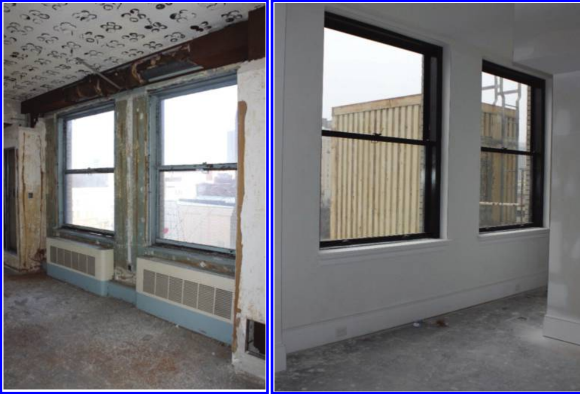
FIGURE 16: Before and after photographs of historic plaster walls in the Tower. After photo shows refurbished plaster and steel windows with “invisible” insulating interior storm units.
